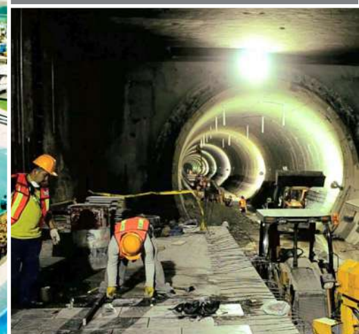
Tunnel Boring Machine, ERA Infra Engineering Limited
