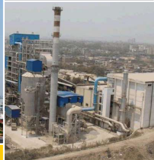
Waste to Energy, New Delhi
